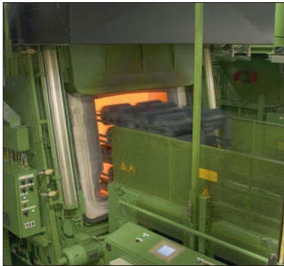
Batch type furnace with controlled atmosphere. Photo: Bodycote Stockholm, Sweden.
